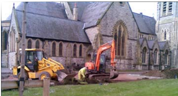
Work began on the car park in April.
